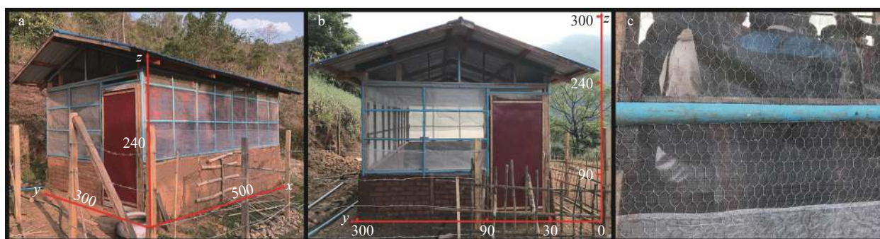
Fig. 3 Low-cost mushroom grow house: a, b measurements of the grow house in cm; c wooden frame covered by insect-proof net and wire mesh.
