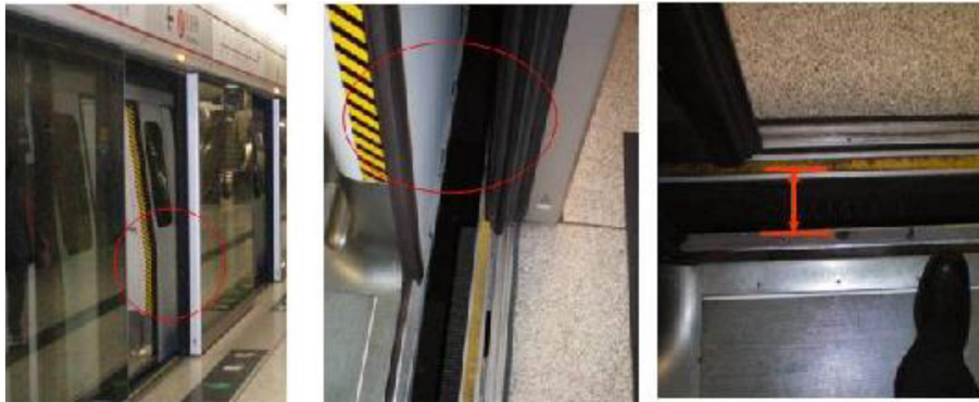
Fig. 1 Images of the gap between PSDs and metro doors.
